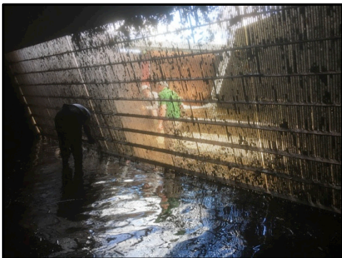
The left hand photograph was taken on the turbine side of the inlet screens, which are cleared of debris each year.
